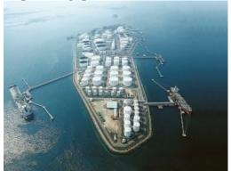
79 tanks for oil products with capacity of 1,037,800 m³ (934 020 tonnes) – planned extension by 216,000 m³ (194 400 tonnes)
